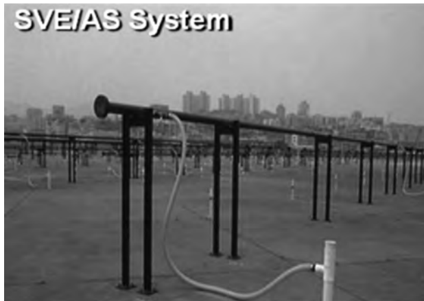
Figure 1 - In-situ Soil vapor extraction in couple with air sparging for both unsaturated soil and saturated soil
