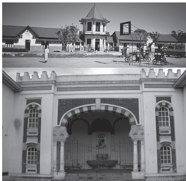
Figure 1. Building of the Antsirabe thermae; outside views
