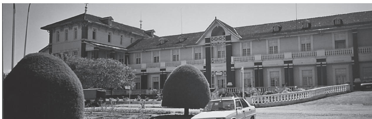
Figure 3. The thermae Grand Hotel; view from outside
