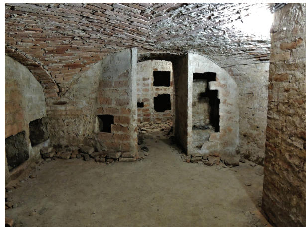
Figure 1. View of the second room of the crypt: the openings on the cell walls show the inner step on which are visible the remains. In the upper portion of the walls, some inscriptions can be clearly read on the remaining plaster.
