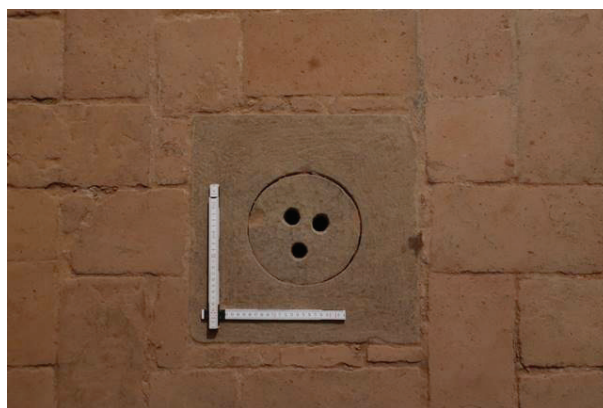
Figure 4. Central drainage pit on the floor of the sepulchre.
